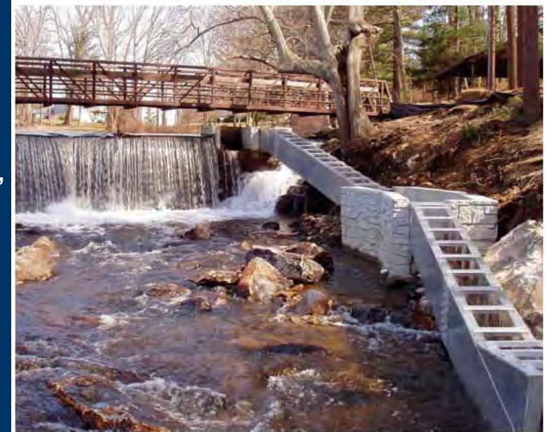
Fish Ladder at Jordan Mill Pond, Waterford, Connecticut, created using settlement funds from the RTC 380 oil spill.
